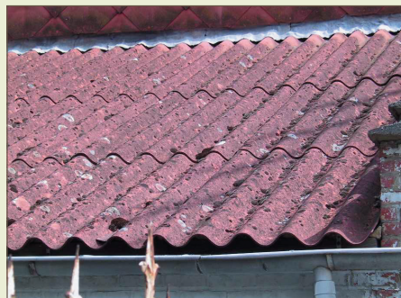
Dakgolfplaten in asbestcement
