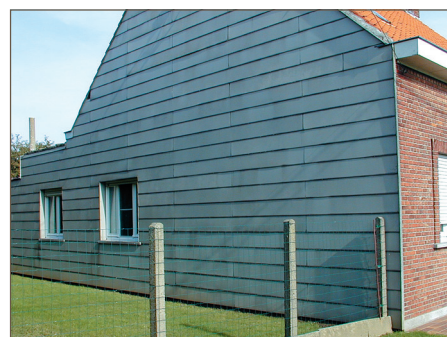
Gevelbekleding in asbestcement
